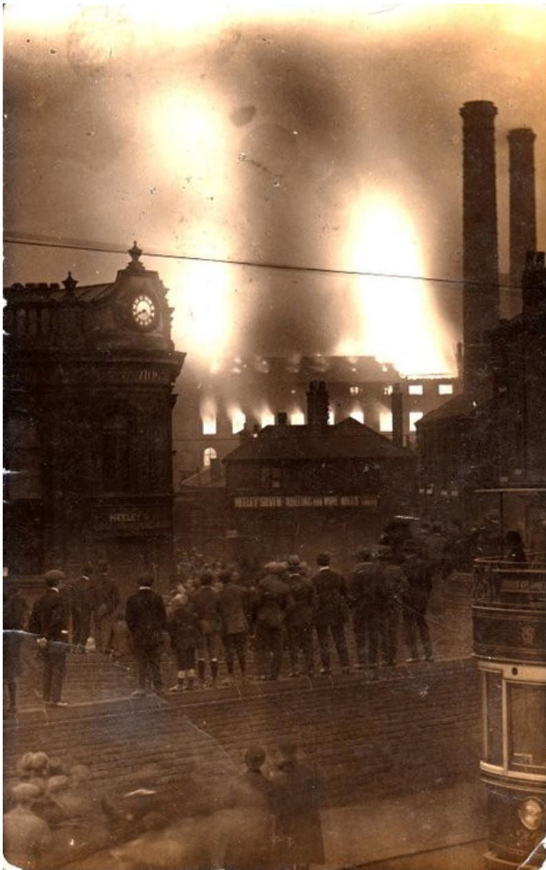
Fire at Messrs. C.T. Skelton, Sheaf Bank Work's, Heeley, 23rd April 1921
